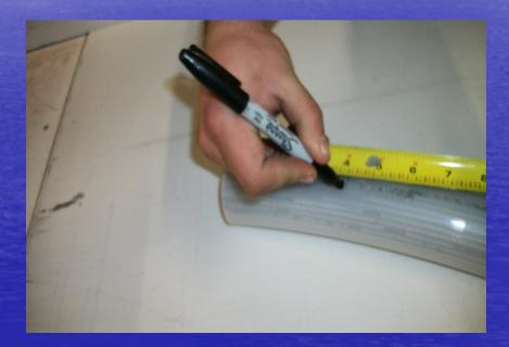
Place the pipe stripper on the Co-Flex pipe with the blade away from the end of the pipe.
