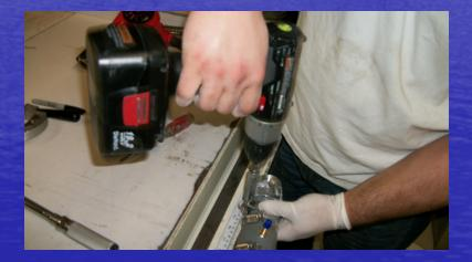
Tighten slowly, moving the screw gun back and forth. This prevents pinching of the pipe. Do not over tighten at this point. Allow lube bonder to set for 1 hour.
