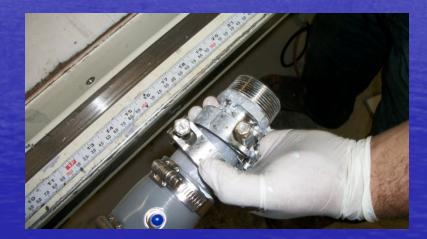
Place the 1st clamp 1/4" from the end of the Co-Flex pipe.
