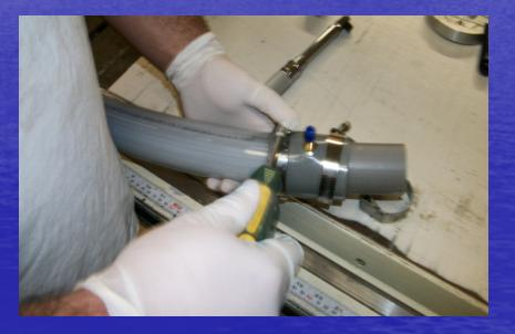
Spray the inside of pipe clamps with white lithium grease. Spray the bolt also. Place the pipe clamps onto the pipe with the bolts in opposite directions.
