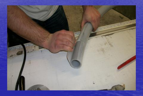
Place test boot (if required) over the pipe first.
