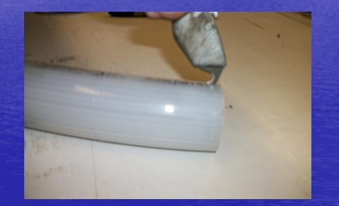
Tear off the outer secondary at the 4" mark.
